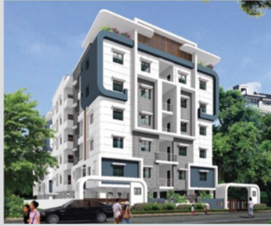
Green Fort, Fort Road, Warangal
